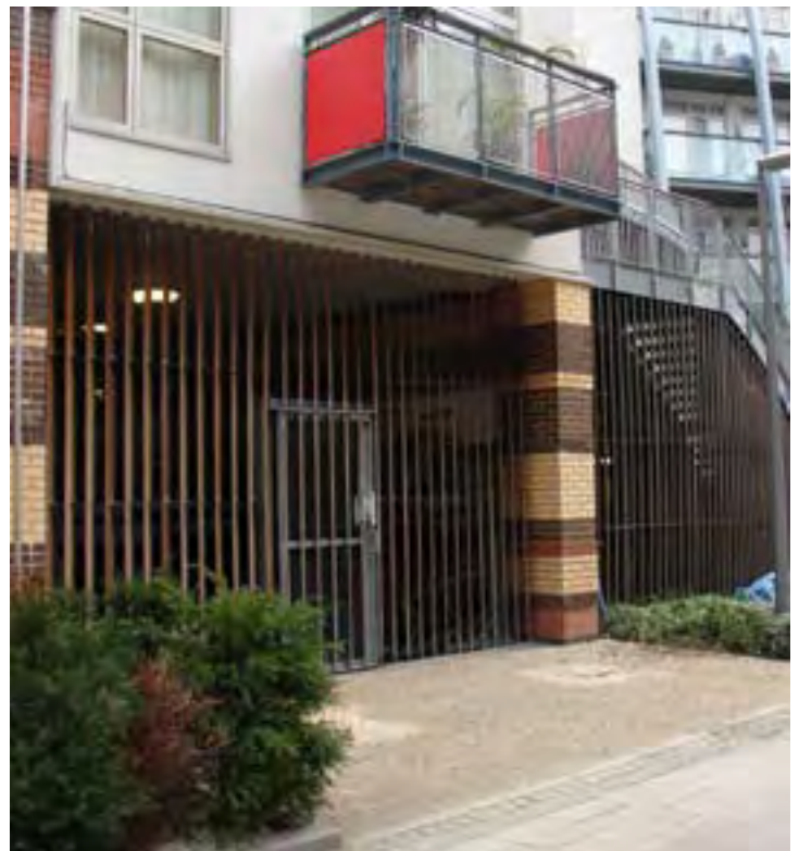
INTEGRATED CYCLE STORAGE BEHIND LOUVRED ENCLOSURE
